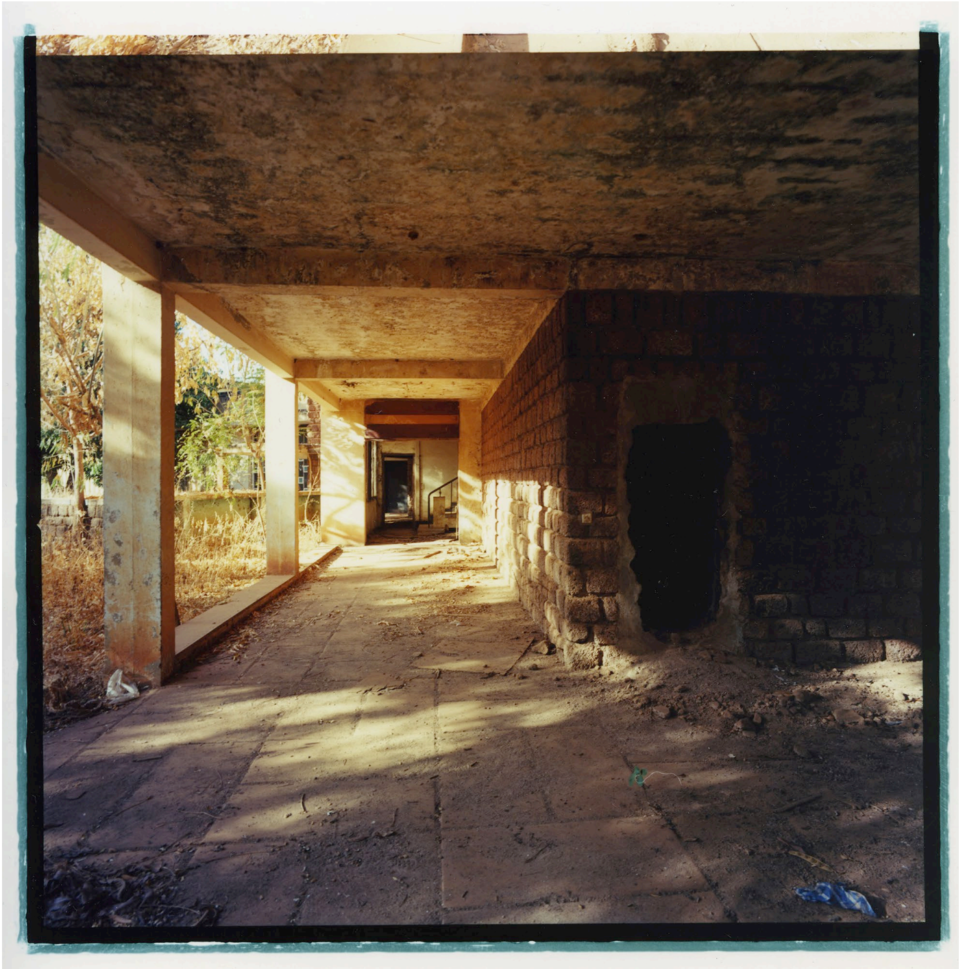
Former Embassy buildings behind the Thomas Sankara Memorial, Ouagadougou, Burkina Faso, 2022
